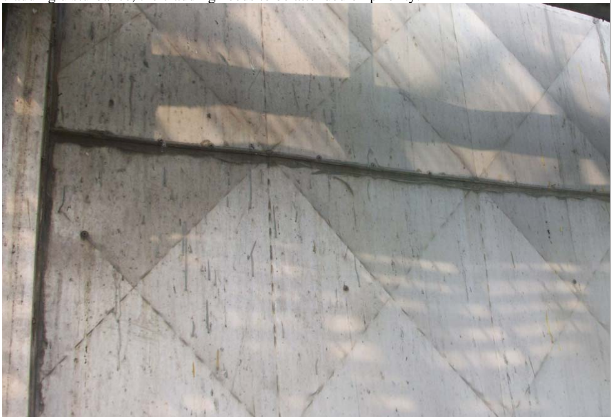
Photo 19: In outdoor installations, sealant shall be used at the cladding sheet joints. This ensures, the rain water does not go inside the insulation.
